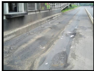
Figure 5 Typical failures in the area of bus shelter
